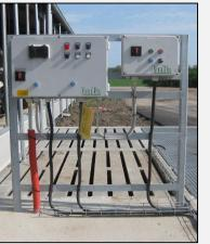
PLC control systems can be fitted with temperature sensors, pressure sensors, frequency converter, logbook, and remote monitoring.
